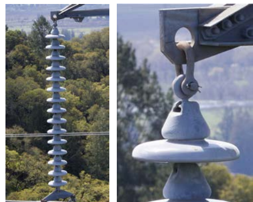
Views of a transmission insulator made possible by high-resolution imagery
